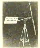
★ Charger for six volt batteries. Propeller automatically adjusis self to wind conditions—speed control safeguards generator from overload. Cut-out prevents overcharging. Animeter shows rate of charge. Mounts atop barn or house. Special co-operative price of \$10 to purchasers of Crosley battery radios. Ace Products Corp., Cincinnati, Ohio— RADIO TODAX
