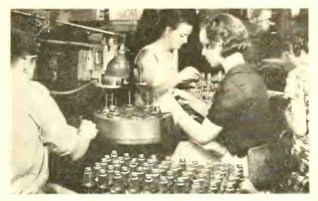
Welding metal-tube shells in the Raytheon factory. The complete assemblies are placed upside down in the rotating welder table.
